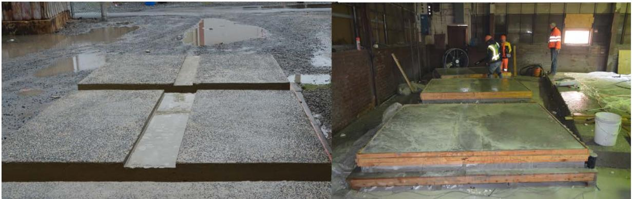
Figure 3. Mockup slabs before and after placing UHPC
