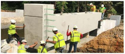
concrete variable height stub abutments. Two separate sections were cast for each abutment. Both abutments were able to be set in just over an hour. A closure pour consisting of Type I 4,500 psi concrete with a 2% high early strength admixture was used to connect the piles to the abutments. By using this concrete mix for the closure pour, the contractor was able to place the beams one day after performing the closure pour.
