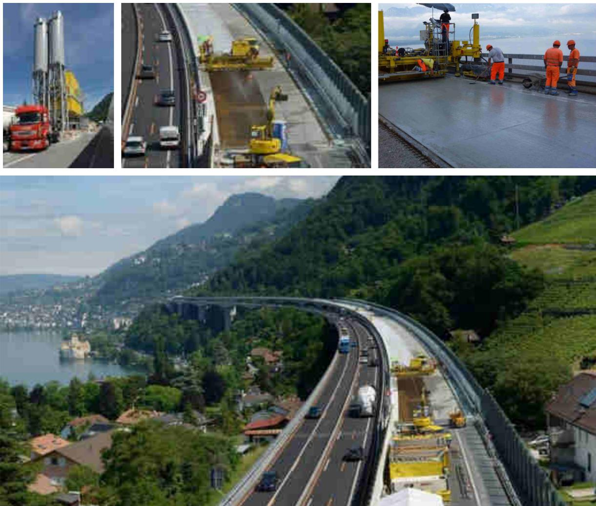
**Figure 11. Implementation of thixotropic Ductal® on Chillon viaduct's deck**
