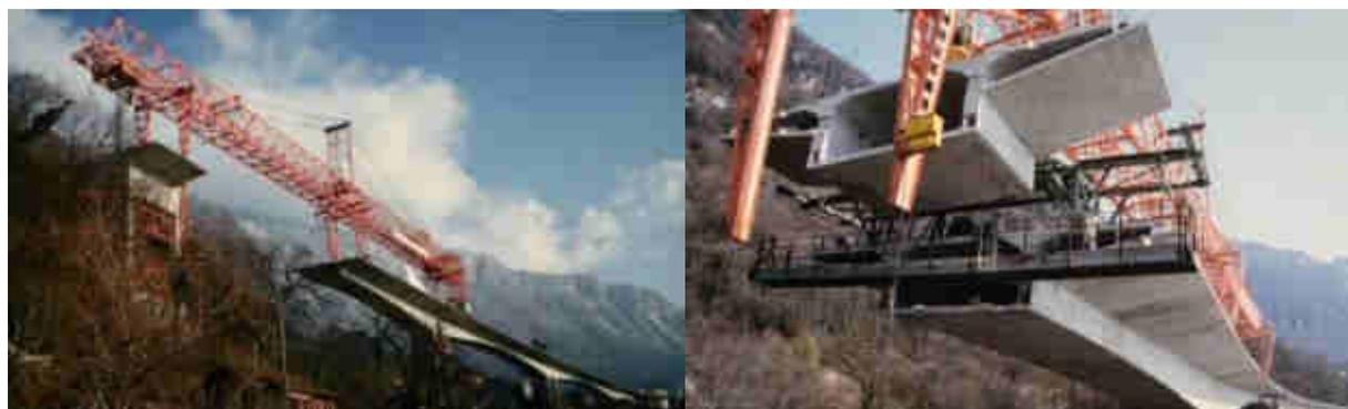
**Figure 2. Construction of the viaduct with prestressed box girder segments**
