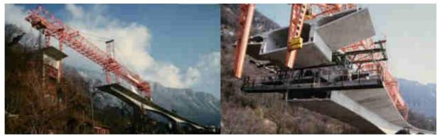
Figure 2. Construction of the viaduct with prestressed box girder segments
