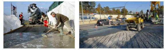
Figure 5. Examples of applications with strain-hardening UHPFRC
