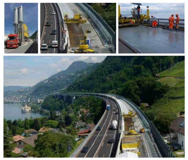
Figure 11. Implementation of thixotropic Ductal<sup>®</sup> on Chillon viaduct's deck
