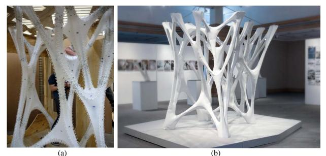
Figure 3. (a) Formwork during assembly; (b) Final prototype after formwork was removed
