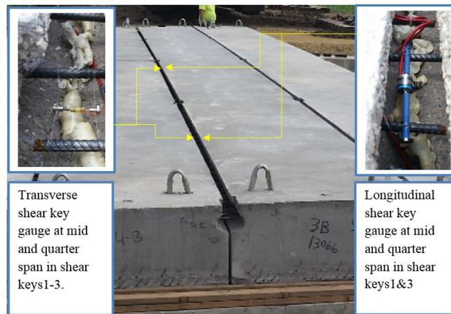
**Figure 5. Transverse and Longitudinal Shear Key Gauge**
