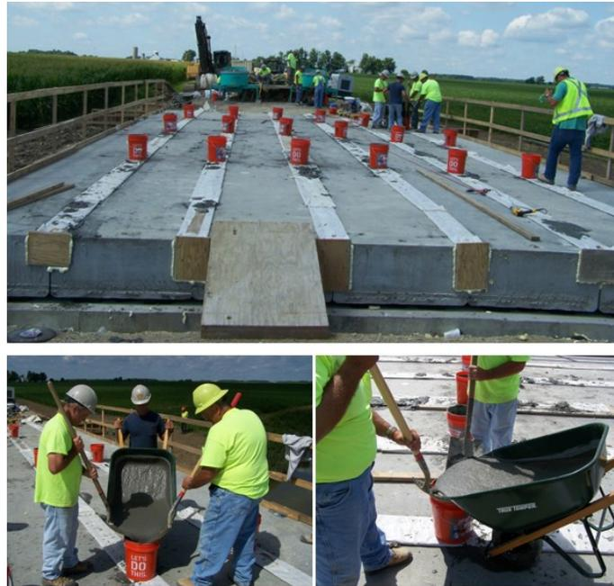
**Figure 6. Placement of UHPC into the Longitudinal Shear Keys**
