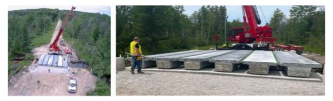
Figure 2: Construction process of the UHPC/PBTG bridge system
