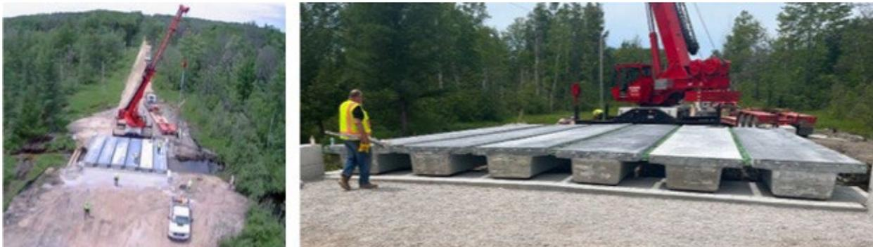
**Figure 2:** Construction process of the UHPC/PBTG bridge system
