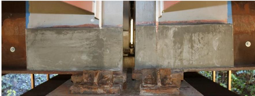
**Figure 1. Completed beam end repair in East Hartford, CT.**
