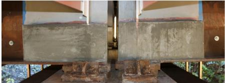
Figure 1. Completed beam end repair in East Hartford, CT.
