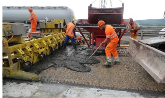
**Figure 6: Preliminary UHPC placement before thickness equalization by the finisher**
