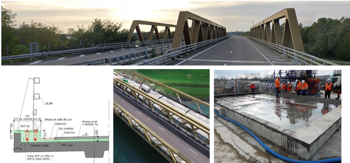
**Figure 1: UHPC overlay on the Warren-type A36 bridge, substituting top of the concrete slab and ensuring waterproofing as tested on a dedicated mockup.**
