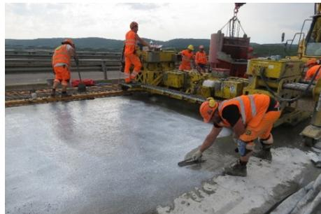
**Figure 8: Simultaneous manual operations for UHPC placement before and beyond the finisher**
