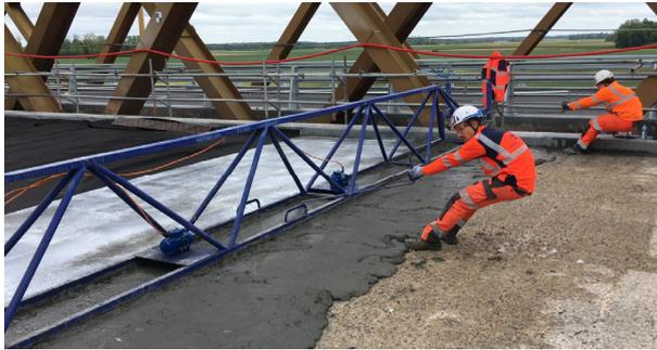
**Figure 5: UHPC overlay extrusion with hand-drawn vibrating screed**
