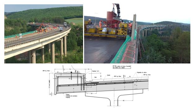
Figure 2: UHPC overlay on the Pont d'Ouche multi-span prestressed concrete girder twin bridges, ensuring waterproofing, surface protection and structural reinforcement for safety barrier anchoring.
