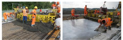
Figure 8: Simultaneous manual operations for UHPC placement before and beyond the finisher
