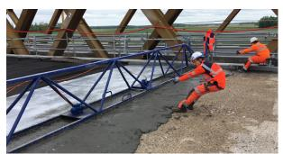
Figure 5: UHPC overlay extrusion with hand-drawn vibrating screed
