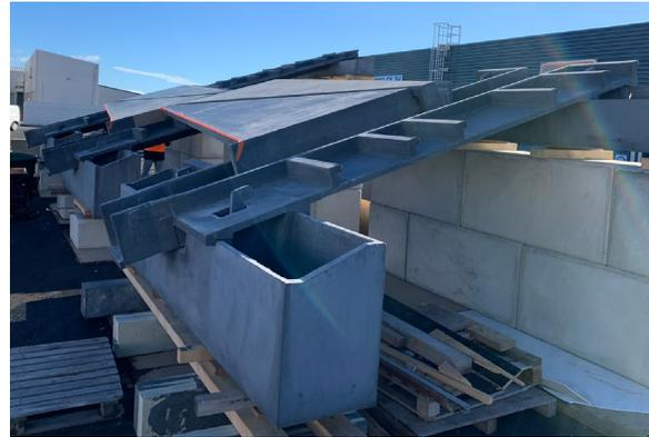
Figure 7: Assembling details: tiles fitted to channel elements, channel elements retained by hooks of the boxes
