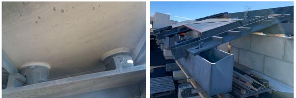
Figure 7: Assembling details: tiles fitted to channel elements, channel elements retained by hooks of the boxes
