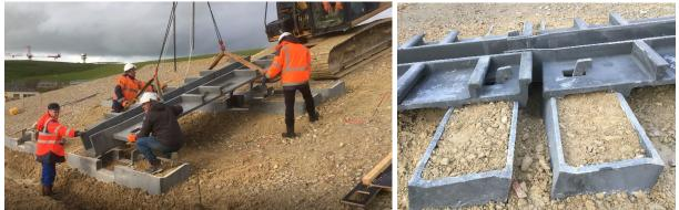
Figure 10: Demonstrator installation: ballasted boxes, handling of the channel element, retaining hooks
