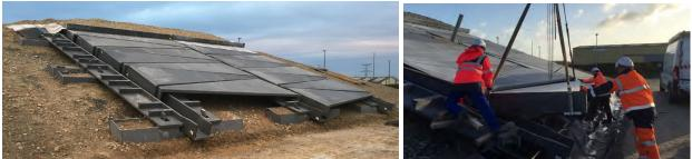
Figure 11: Demonstrator installation: handling, orienting and fitting the single missing tile
