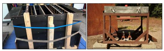
Figure 3. Framework before concrete casting
