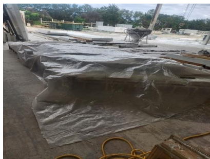
Figure 12. The filled and covered mold
