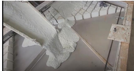
Figure 11. Pouring behind the leading edge
