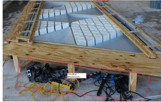
Figure 4. Vibrating attachments under the mold
