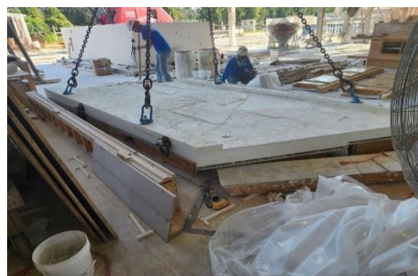
Figure 13. Stripping the panel
