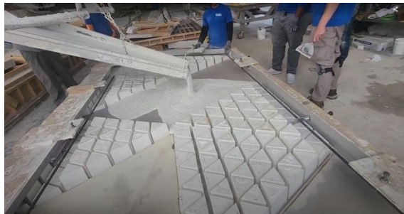
Figure 10. Discharging the UHPC mix
