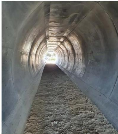
**Figure 1: General view of the ended reinforced Corrugated Steel Pipe**
