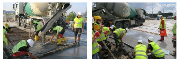
Fig. 6 UHPC casting
