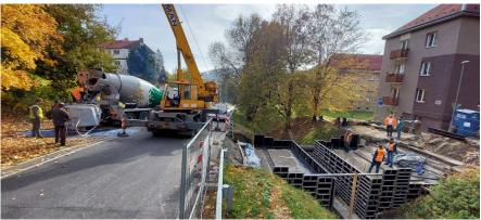
Fig. 1 UHPC casting
