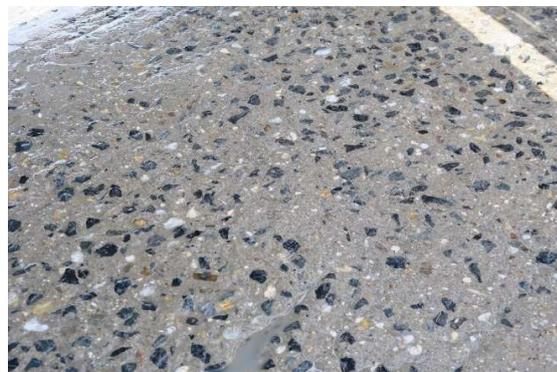
**Fig. 5** Milled concrete surface
