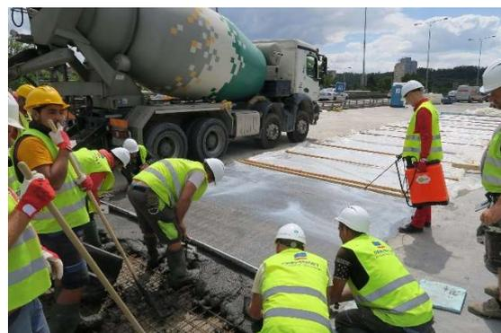
**Fig. 7** UHPC curing
