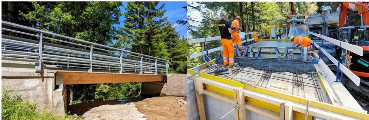
Figure 2 Presentation of the Fruttli Bridge and casting of the UHPFRC deck slab.
