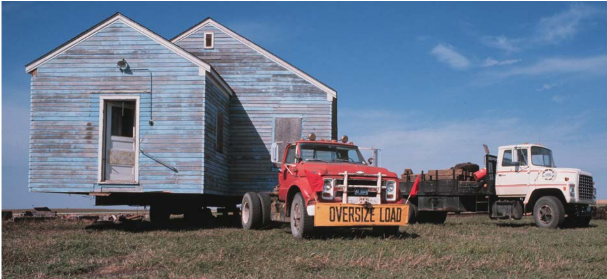
The Cornwell home is loaded on a rig of steel beams and wheels for its move from the farm to the town of Rolfe. 1989.
