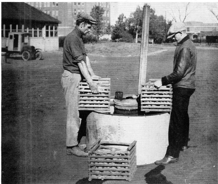
Treating seed potatoes with hot formaldehyde, a process devised by I. E. Melhus at Iowa State College, did in one minute what it formerly had taken four hours to do in whipping fungi attacking the tubers.—CHAPTER 6, WINNING THE FIGHT AGAINST PLANT DISEASES.
