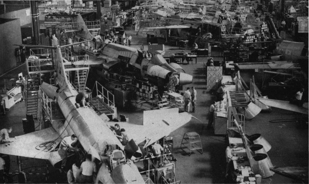
The production line at an aircraft plant shows several twin jet fighters being fabricated in the final assembly area. In addition to planning and designing the aircraft, the engineer supervises its manufacture. (Courtesy McDonnell Aircraft Co.)
