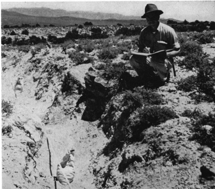
The mining engineer directs the field work of exploring and sampling a new prospect. Here he is shown mapping the surface geology exposed in the trench. He may stay to construct and operate the mine, or he may move on to a new field.
