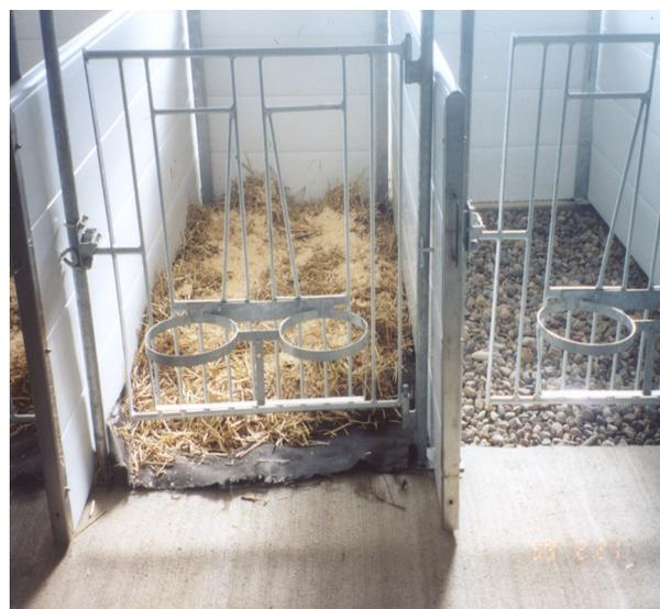
Figure 2. Straw is on geotextile above pea gravel.
