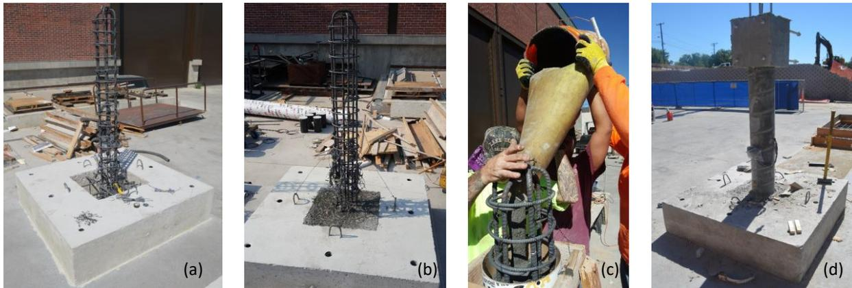
Figure 2. Specimen Construction Stages: (a) Casting of NSC Footing; (b) Casting of UHPC Footing; (c) Casting of UHPC Column; (d) Casting of UHPC Column Head.
