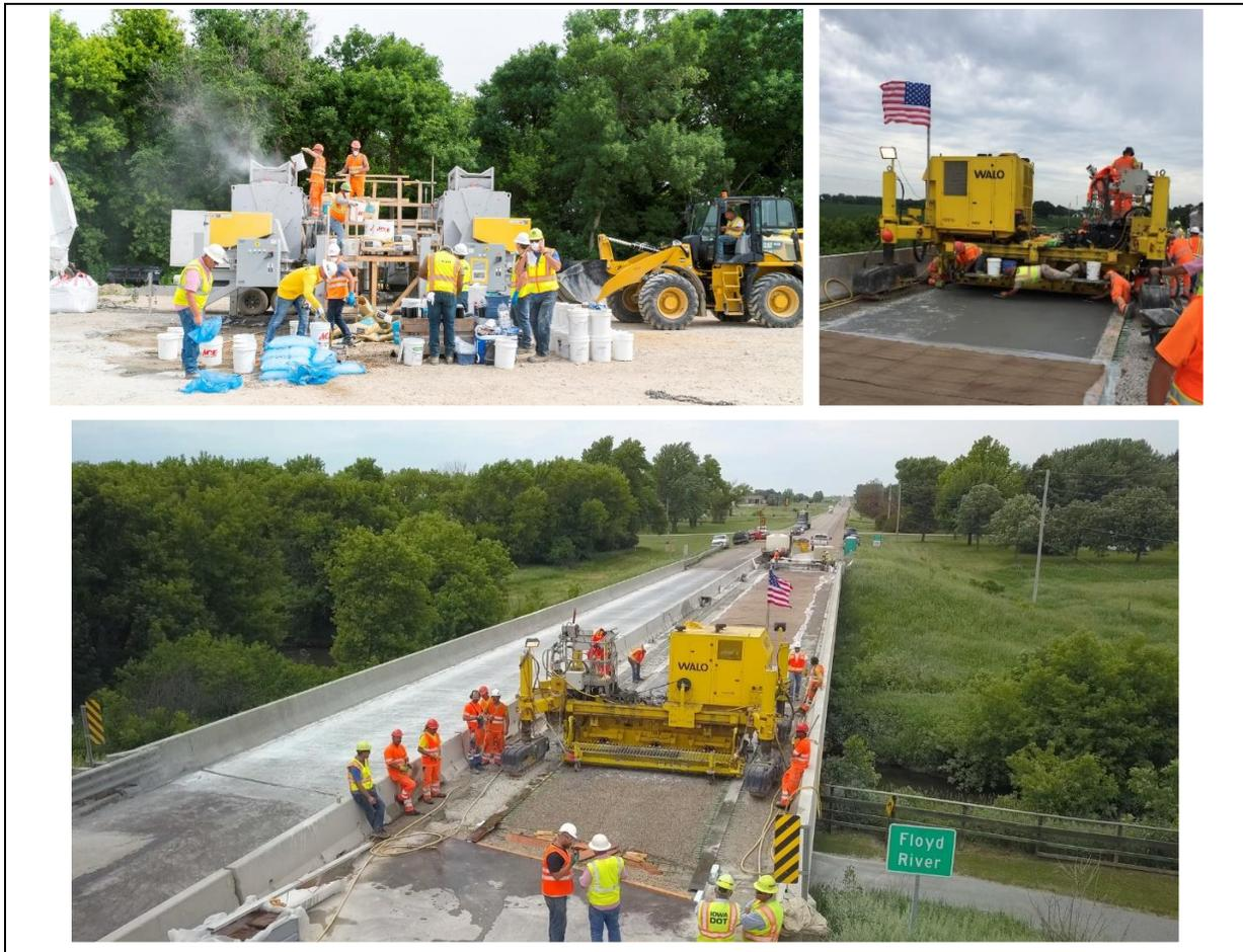
**Figure 1. UHPC Installation with paving machine**
