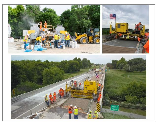
Figure 1. UHPC Installation with paving machine
