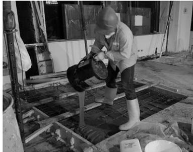
a) Reinforcement slab casted on site.
