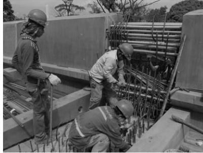
**Figure 13. Preparing segment above the pillar for casting.**
