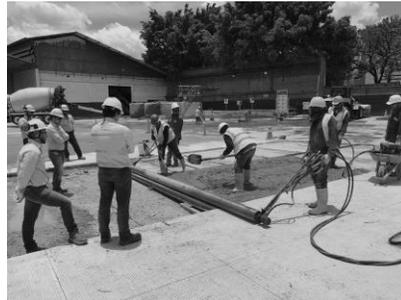
**Figure 14. Overlay placing.**
