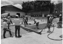
Figure 14. Overlay placing.
