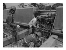
Figure 13. Preparing segment above the pillar for casting.
