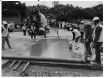
a.). UHPC overlay, Argos Concret plant.
