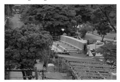
Figure 9. EAFIT footbridge plywood decks and scaffolding process.
