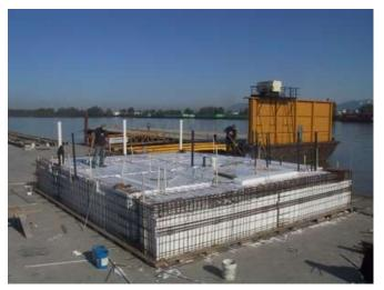
Figure 1 - Concrete Floating Foundation with EPS Foam (Jostrom, 2013)
