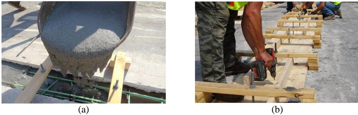
**Figure 7 Casting of UHPC into a joint between beams: (a) placement; and (b) top forms installed**
