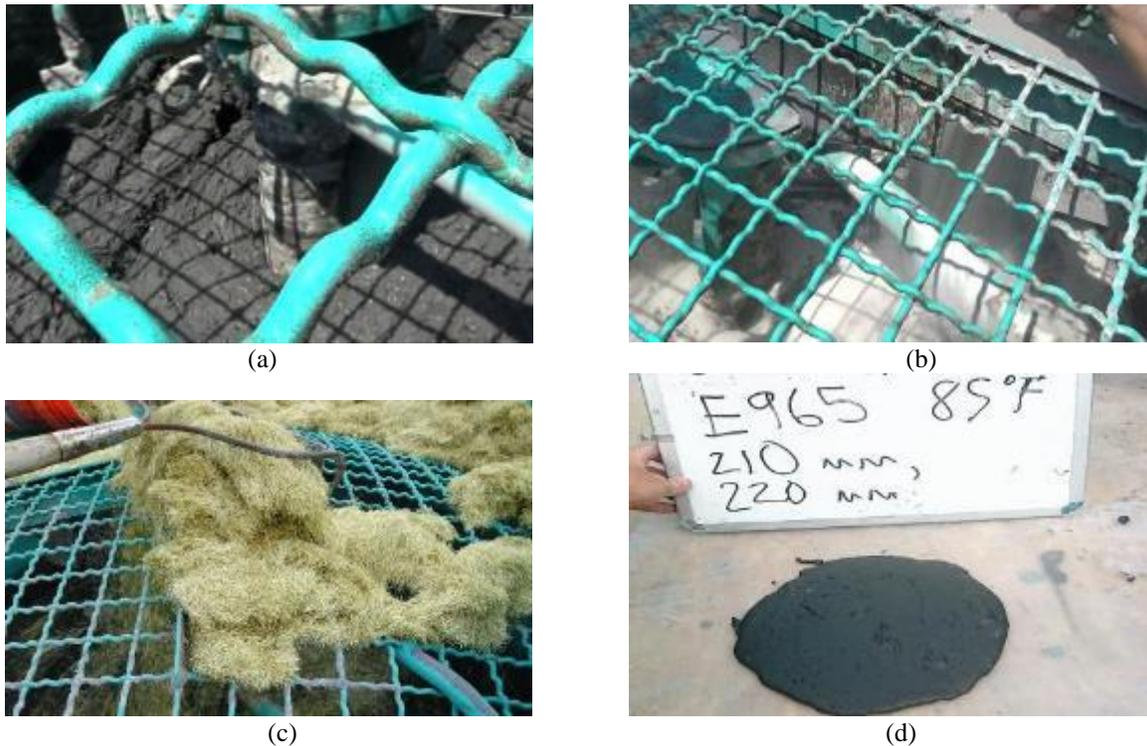
**Fig. 6 Field mixing procedure and testing of UHPC mixture: (a) after turnover, thick slurry is formed; (b) incorporate remaining silica sands and continue mix to disperse and homogenize; (c) addition of steel fibers; and (d) flow test**
