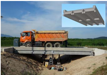
Figure 9. Andong Bridge I ( \pi section)
