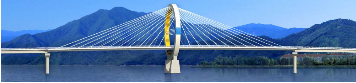
Figure 11. Bird's eye view of LEGOLAND UHPC Cable Stayed Roadway Bridge
