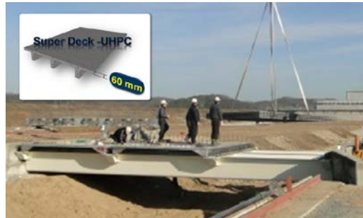
Figure 10. Andong Bridge II (rib deck)
