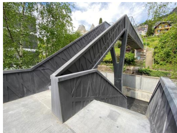
Figure 5 The Chaumény footbridge - Example of very subtle post-tensioned U-shaped segmental bridge with span ca. 22.5 m (73.82 ft.) from Switzerland, figure is taken from Géhin
