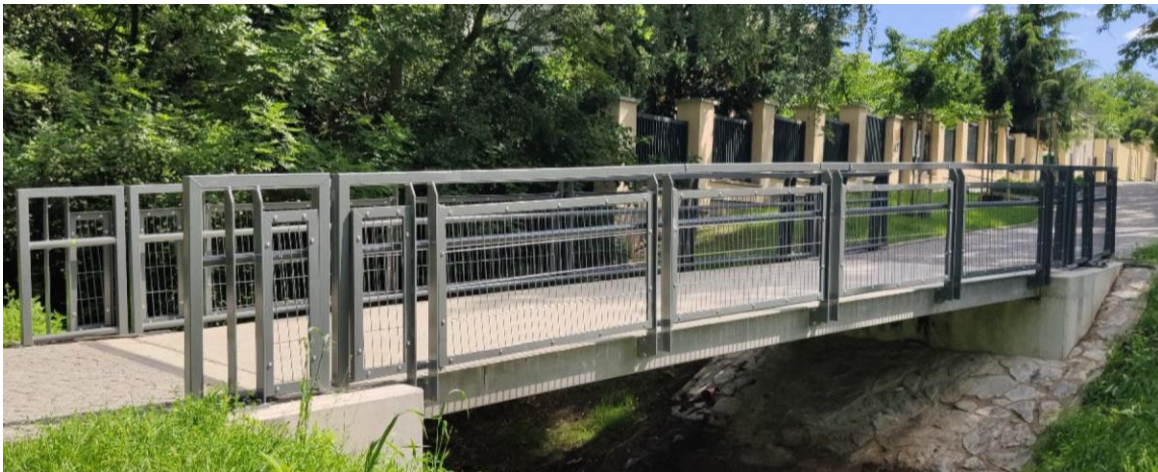
Figure 3 View of the completed footbridge Čelákovice
