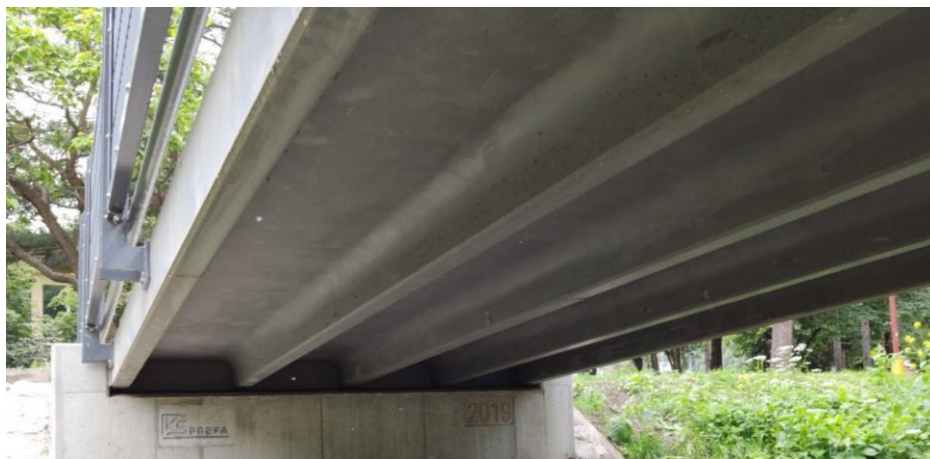
Figure 4 Bottom view of the finished structure of footbridge Čelákovice
