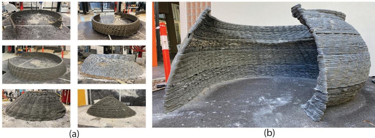
Figure 4 (a) Some of the separately 3D printed sections of the fire shelter (b) Partly assembled fire shelter on-site
