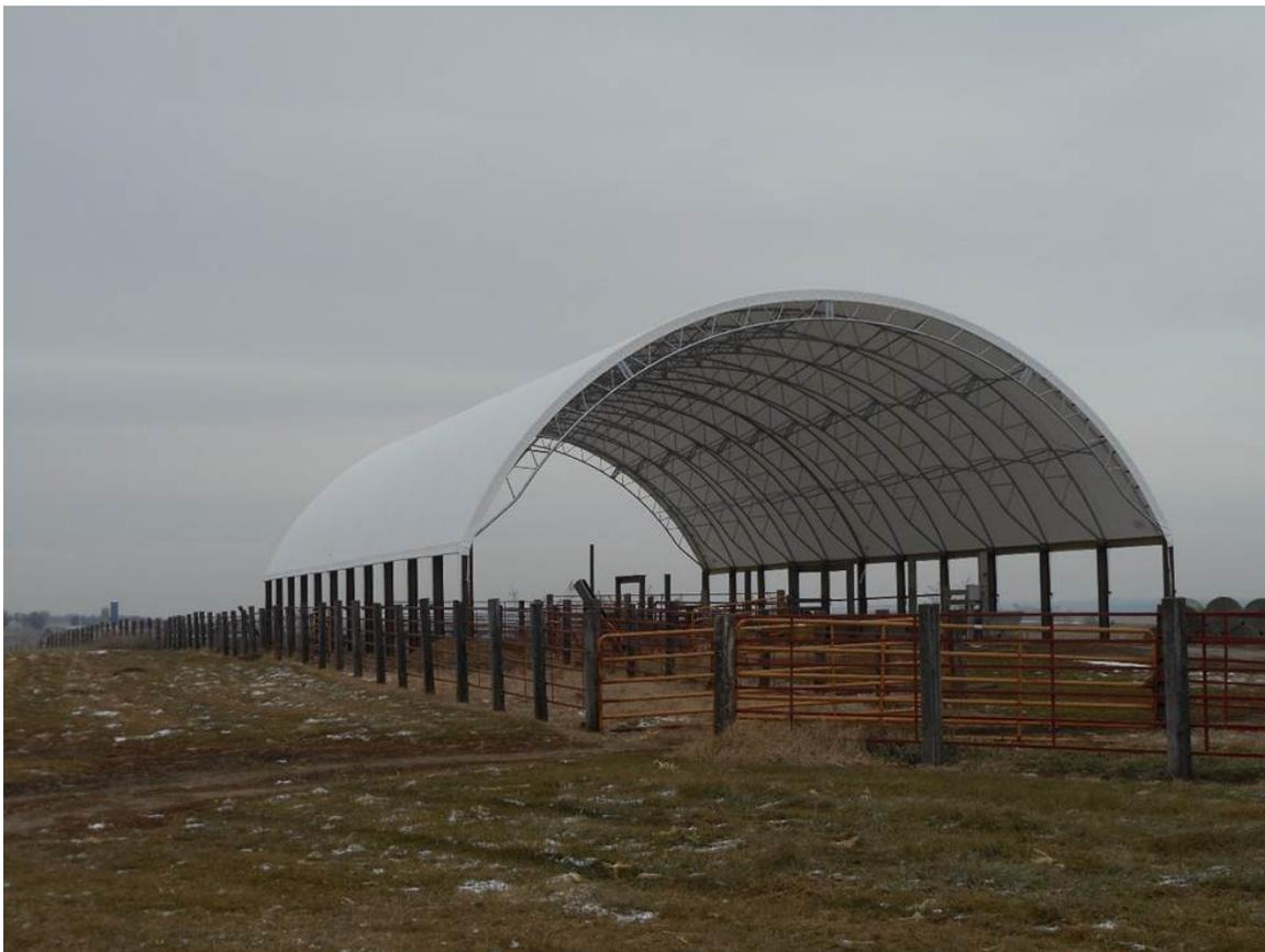
**Figure 1. The revised hoop barn (68 ft x 132 ft) for cattle feeding (not fully finished).**
